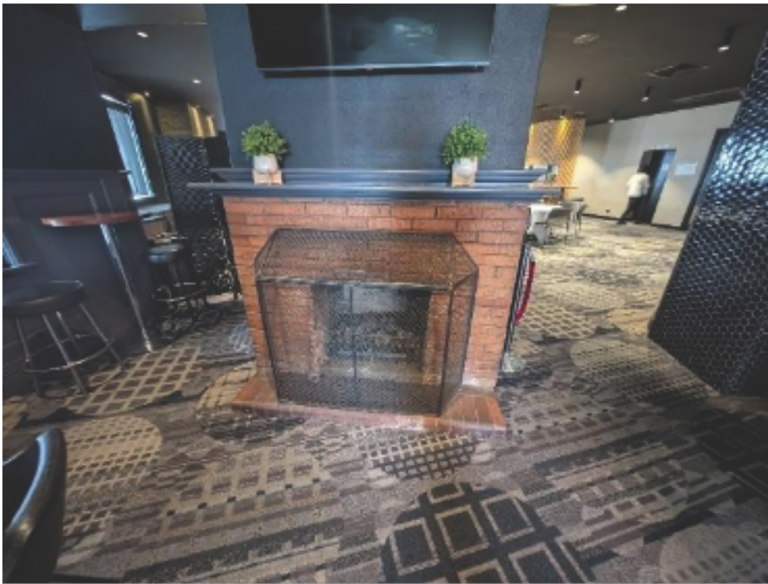
Figure 5. Unused Fireplace Creating Unnecessary Air Exchange
