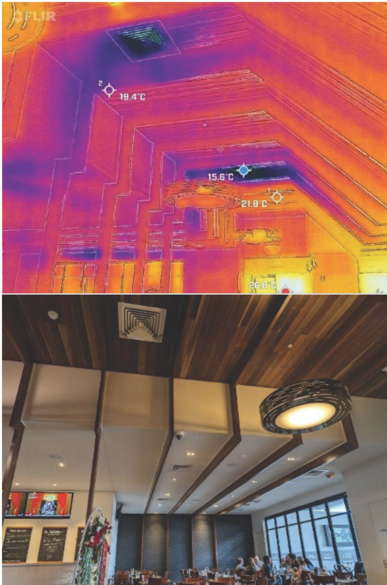
Figure 6. Roof Beams Influencing Air Movement and HVAC Performance
