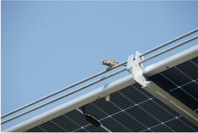
Figure 16. Snow guards are a low-cost way to hold snow while it melts. (Photo credit: David. S. Goldman, used with permission)
