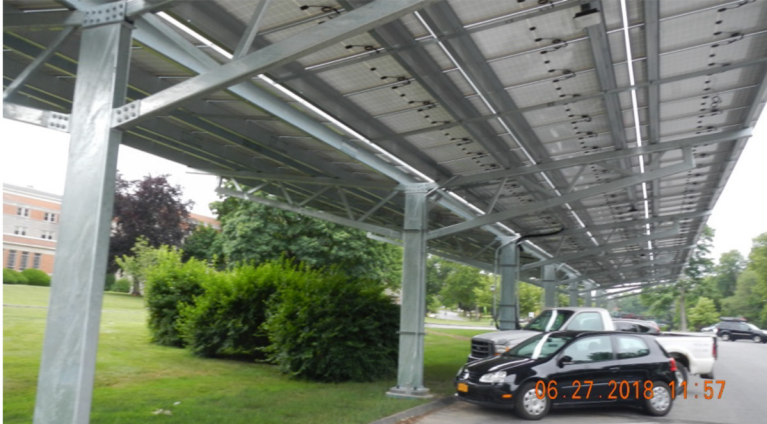
Figure 2. A double-tilt canopy at a college (Photo credit: Lindsay Audin)
