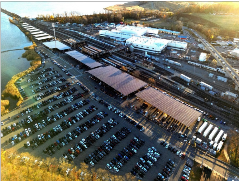
Figure 6. The Croton train station canopy system includes 12 canopies. (Photo credit: Mike Bole, Bow Renewables, used with permission)
