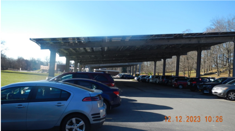
Figure 1. A single-tilt canopy at an elementary school (Photo credit: Lindsay Audin)
