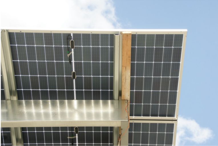
Figure 4. Bi-facial panels have solar cells on the top and underside of a panel. (Photo credit: Lindsay Audin)
