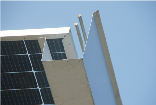
Figure 17. The Croton system includes gutters on the low edges of its canopies. (Photo credit: David. S. Goldman, used with permission)
