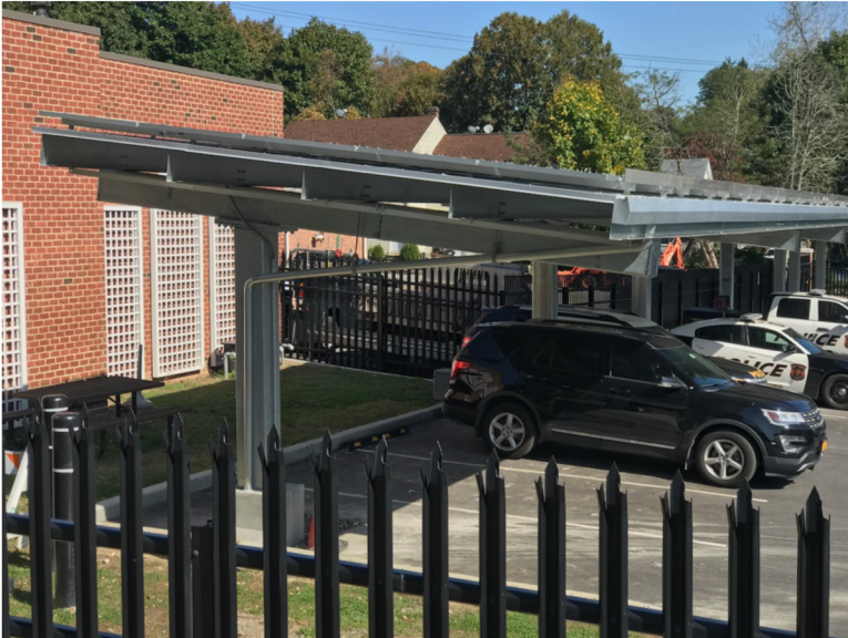
Figure 3. A short-span canopy having one row of pedestals (Photo credit: Leo Wiegman)
