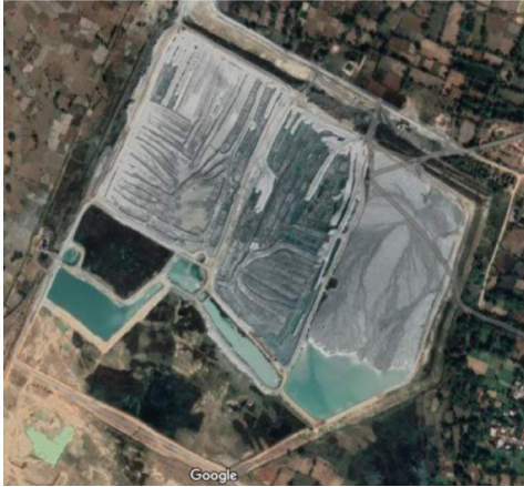
Figure 3. Satellite Image showing ash pond of KTPS, Koderma, JH. (Source: Google Earth)
