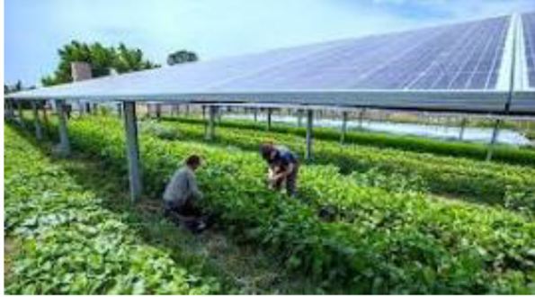
Figure 1. A typical site with simultaneous use of land for agriculture and SPV power
